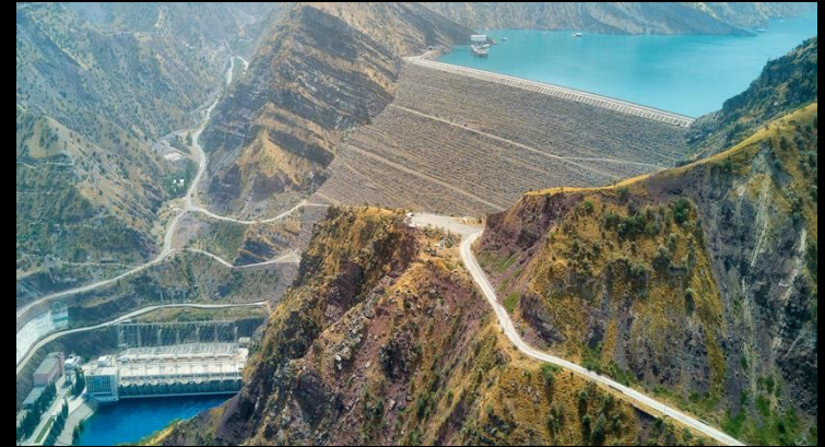
Nurek dam and hydropower rehabilitation, Tajikistan
