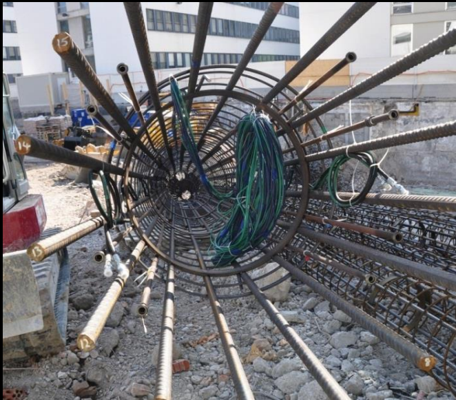
Reinforcement cage prior installation
