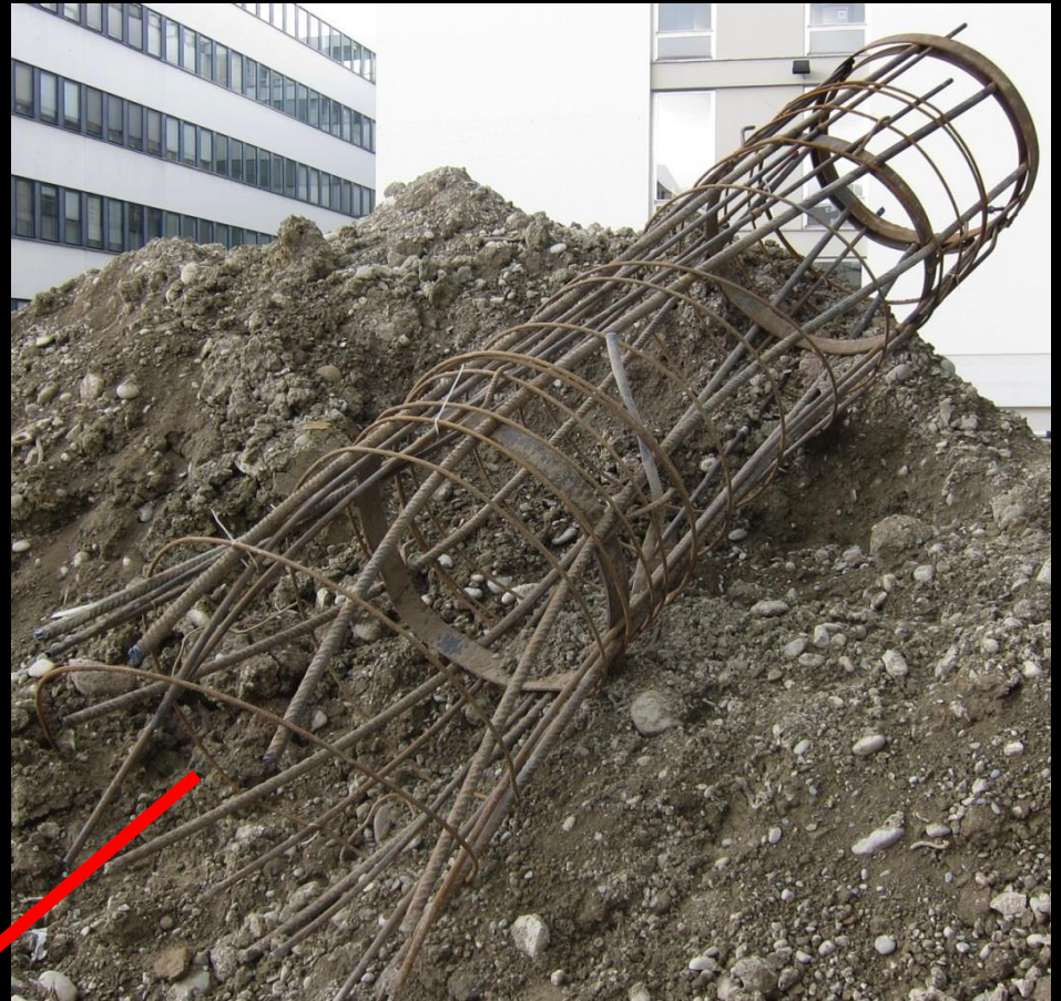
Twisted reinforcement cage after pile dismanteling
