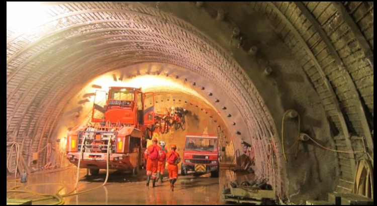
CEVA, Tunnel de Pinchat, Geneva
